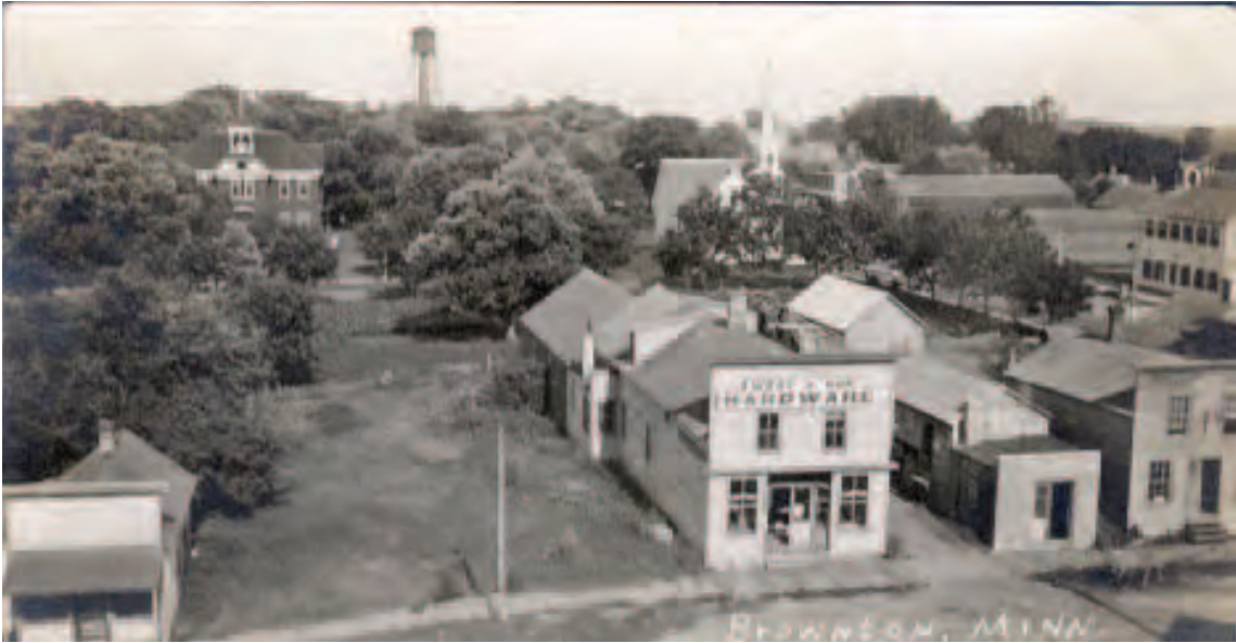
Water tower in background, possibly Division St. in foreground, Brownton, 1900s. Courtesy of LakesnWoods.com.
